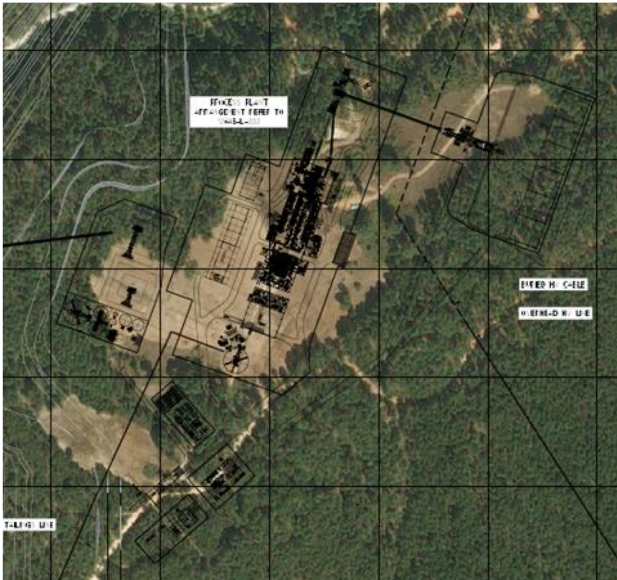
Figure 18.2 Aerial view of the plant site
