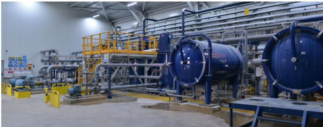
Oxide Processing Plant
